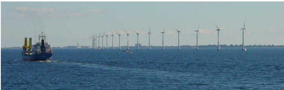
**Figure 7.** The Middelgrunden offshore wind park on Øresund produces 4% of the electricity used in Copenhagen.
